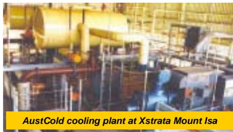
In the evaporator, heat is absorbed into the refrigerant (ammonia) from the secondary coolant (water, brine or glycol). The low-pressure liquid refrigerant, which is at a lower temperature than the secondary coolant, absorbs heat and boils or is evaporated into a gas. In giving up its heat, the secondary coolant can then be circulated to remove heat from the ground, which now
