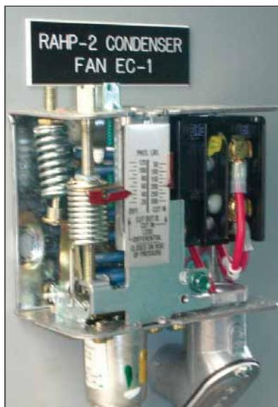
Figure 1: Reverse acting high-pressure controller
