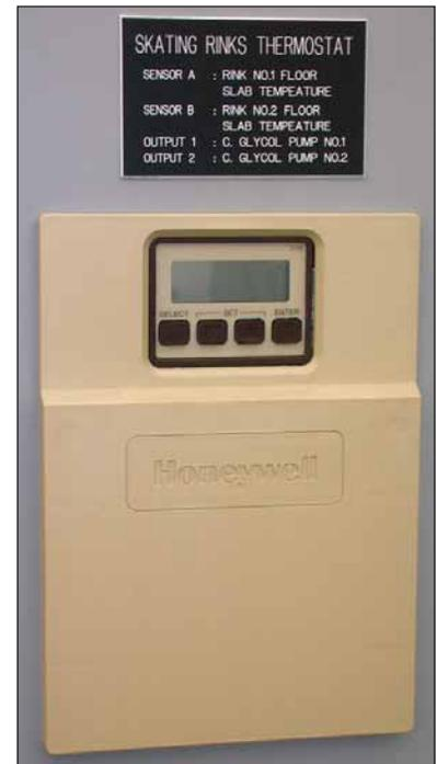
Figure 2: Two-stage slab temperature controller
