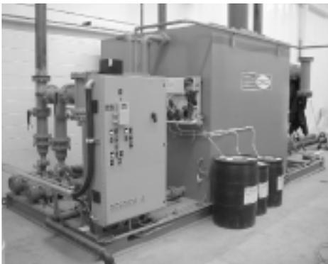
Cimco provides complete pre-assembled packages that minimize on-site assembly and labour costs. Tower water tanks are available with a pre-piped water treatment system, pre-wired and mounted starter and electrical panel, two process pumps and two tower pumps. In addition, tanks are supplied with connections on opposite end of tank for future expansion of the system.
